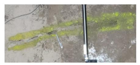
4. Make a mark across the crack with a marker. If the cracks moves in a shearing parallel direction the 2 sides of the mark will move apart from one another and provide valuable information to add to the perpendicular movement recorded by the crackmeter.
