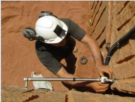
Fig 1: Using d-Conv to monitor a retaining wall
