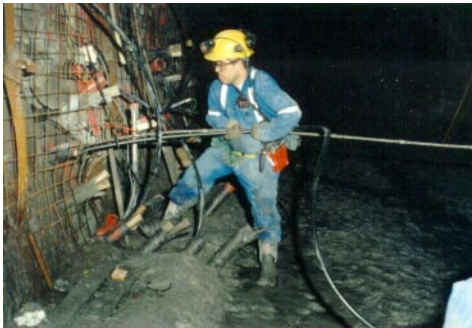
Figure 4: Installing a SMART cable.
