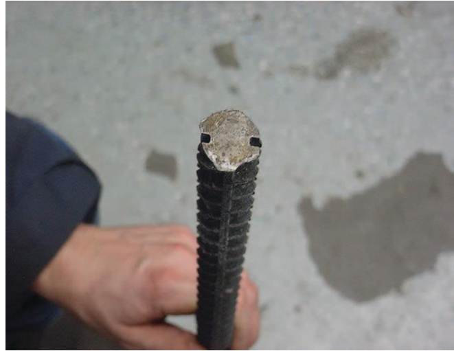
Figure 1. The diametrically opposed grooves cut in the rebar samples.
